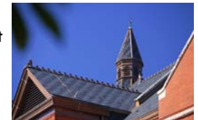
Recycled rubber slate-like tiles are seen on the roof.
