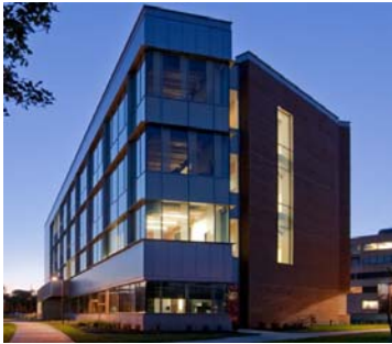
The east elevation of the building.
